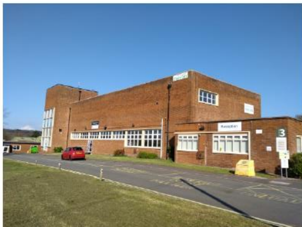
Block 3 Southern and eastern elevations
