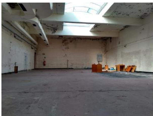
Current internal condition
